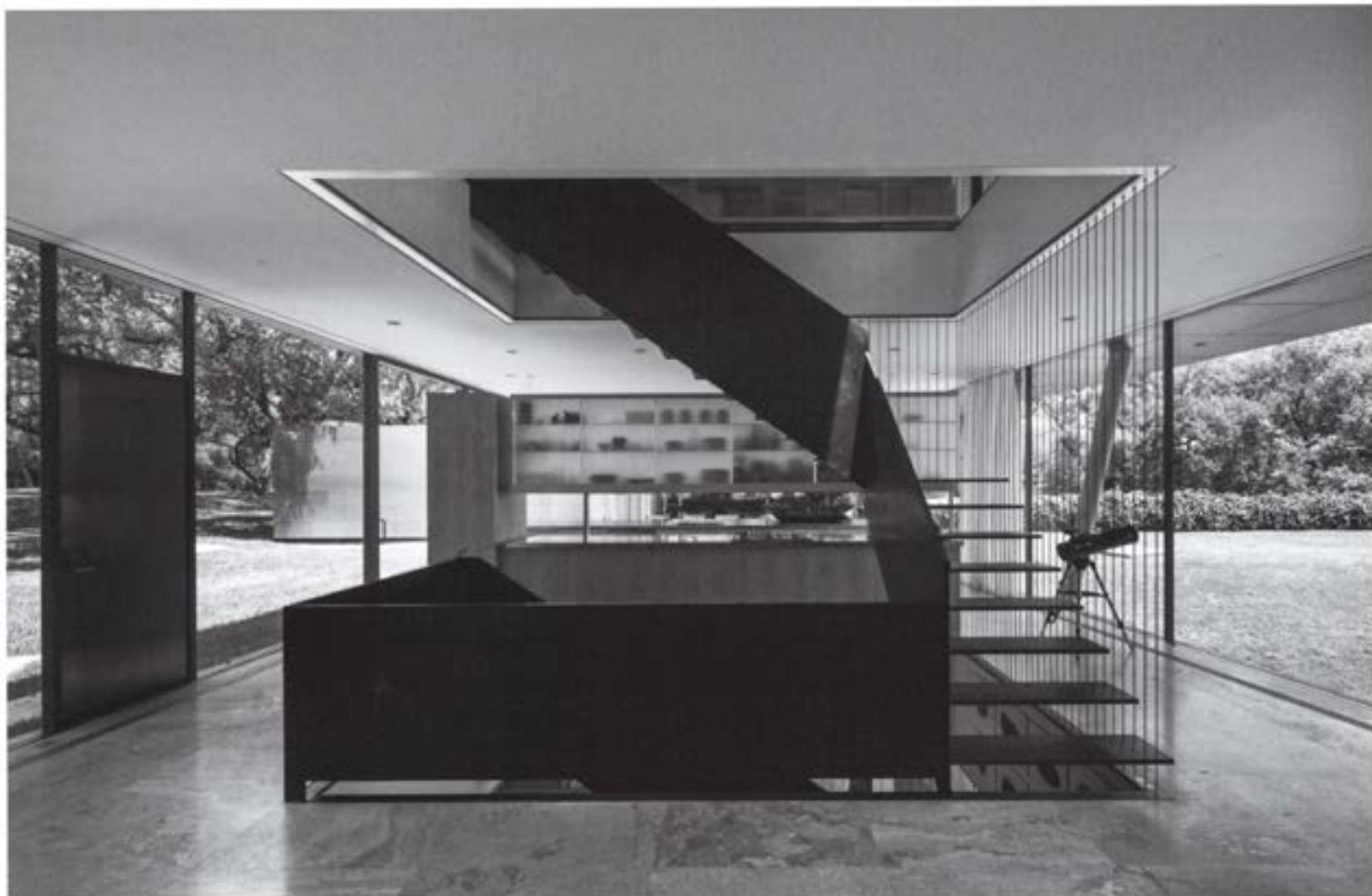
Staircase on ground floor 1階、階段室廻り
