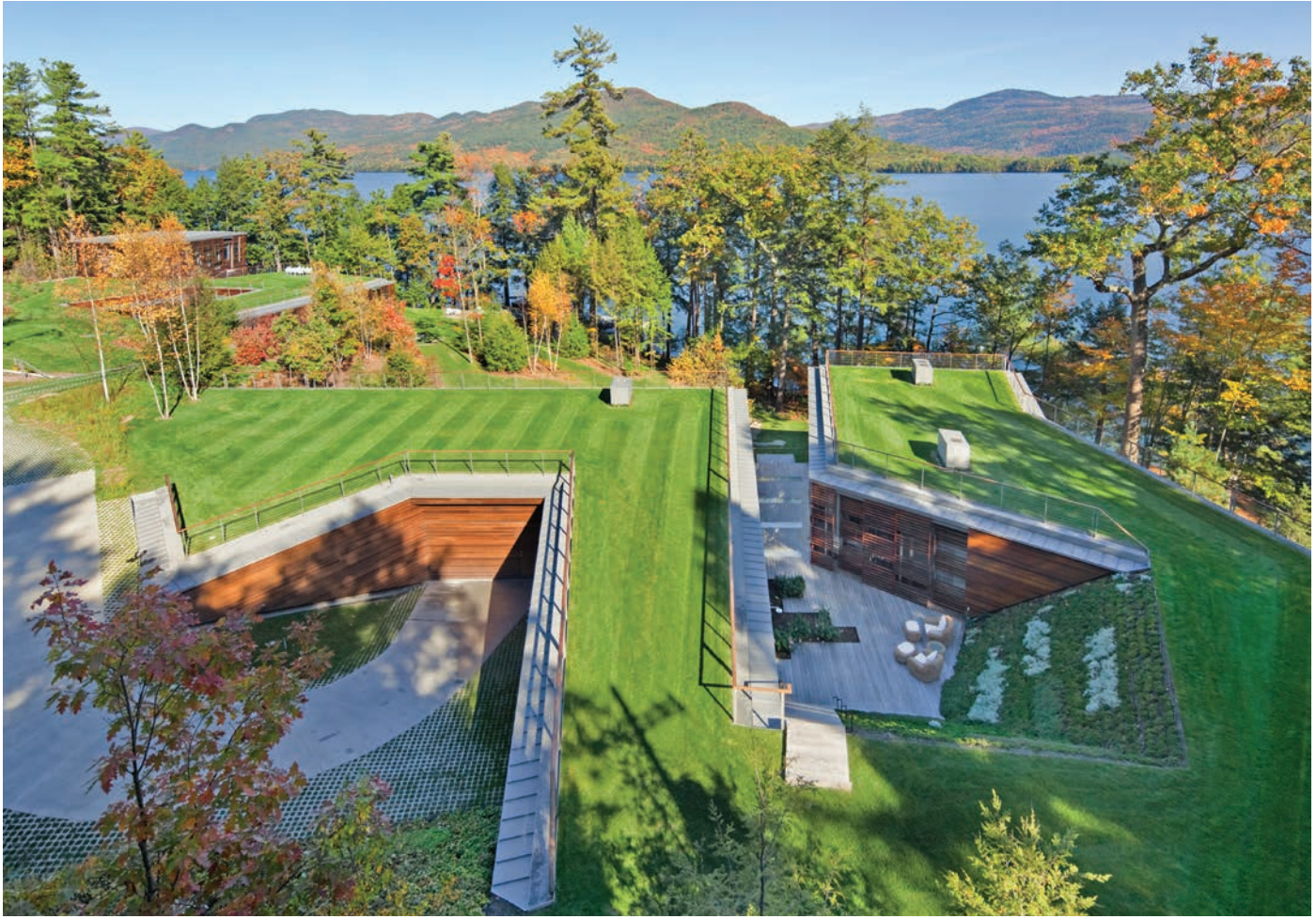
Inspired by the tradition of Adirondack Great Camps, this modern family retreat is nestled into a heavily wooded and steeply sloped lakefront property in Upstate New York.
