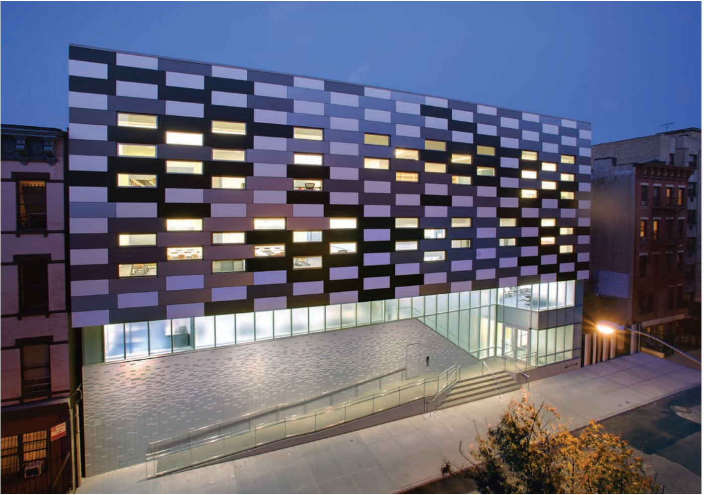
The East Harlem School, a new building for an independent middle school.
