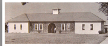
• Boathouse with wing additions
