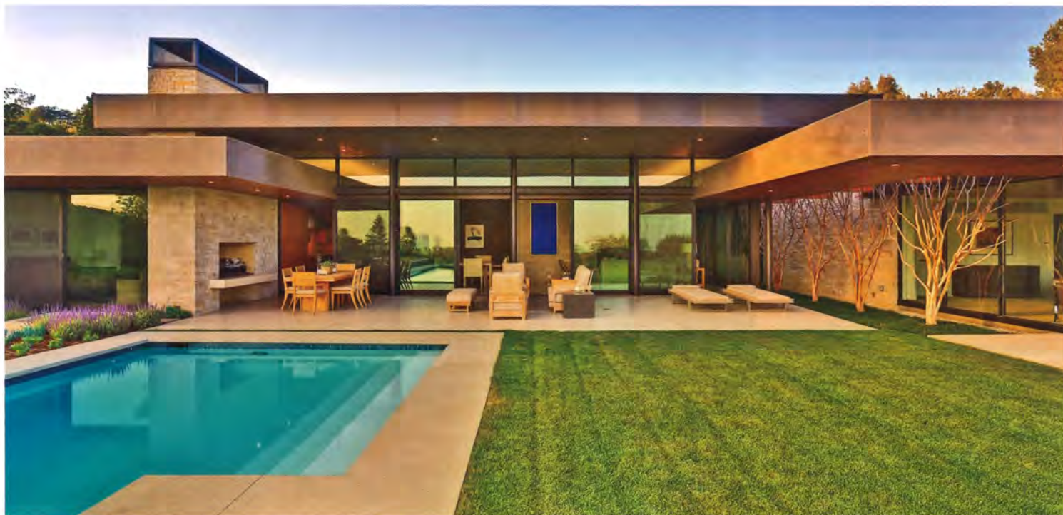
SOUP TO NUTS Among Marmol Radziner’s many design-build projects is a Beverly Hills house for an investment advisor. The firm recently launched a residential-development unit and will do everything from buying the land to marketing the completed houses.
