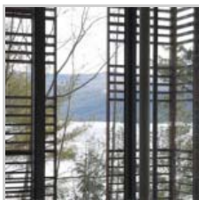
On the second level, the inner screen doubles as a balcony guardrail. (Courtesy GLUCK+)
