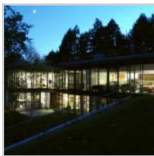
The architects could incorporate large curtain walls without sacrificing efficiency because so much of the buildings’ mass is below-grade. (Courtesy GLUCK+)
