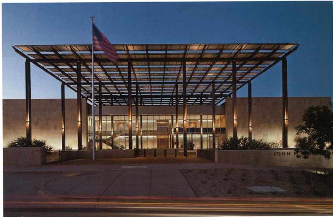
JOHN M. ROLL U.S. COURTHOUSE Ehrlich Architects' $24 million courthouse in Yuma, Arizona, includes photovoltaic panels mounted on a weathered-steel entry canopy that supply 20 percent of the building's electricity.
