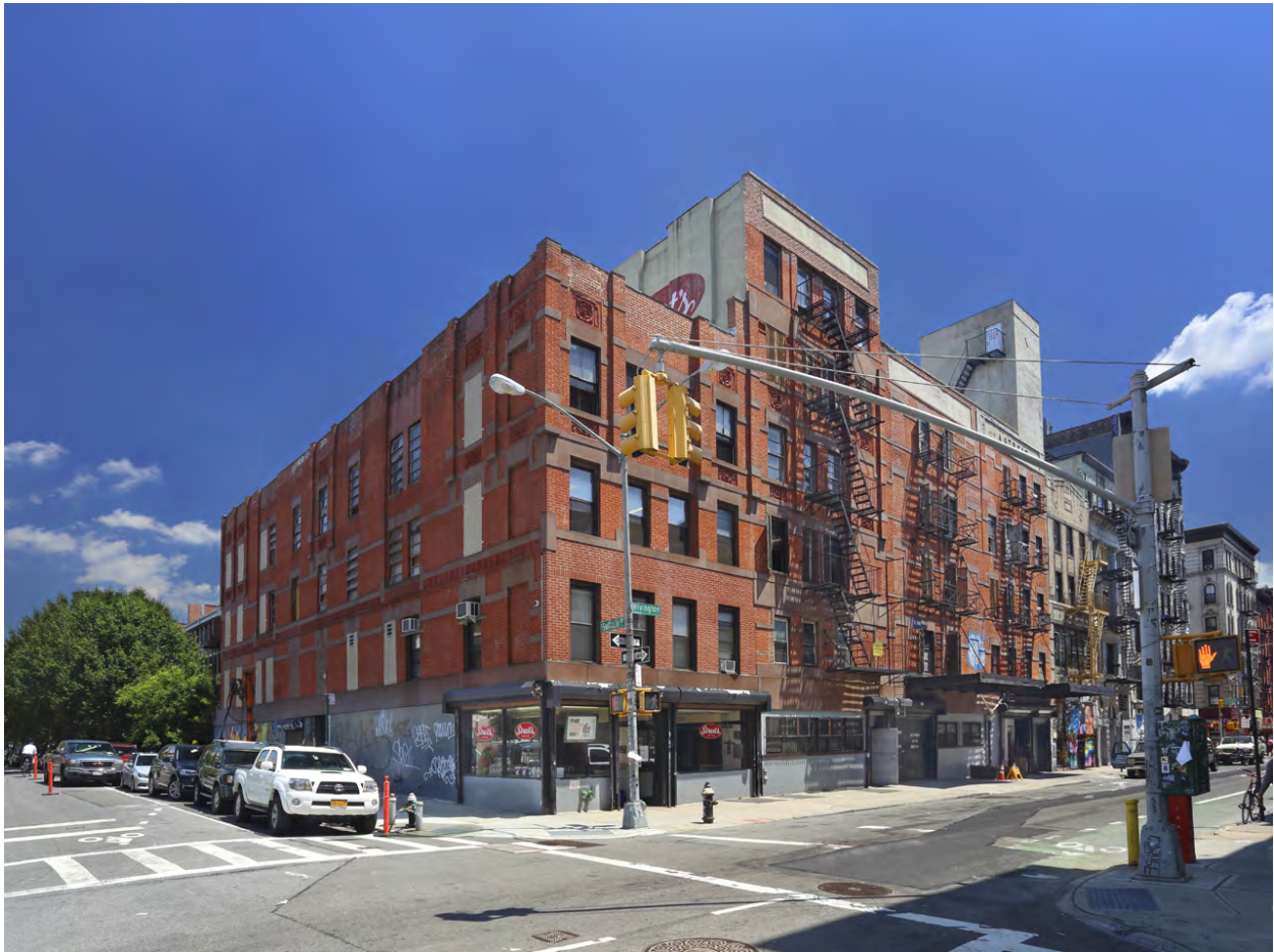
Streit's Matzo Factory prior to demolition. Photo by Richard Sylvares.
