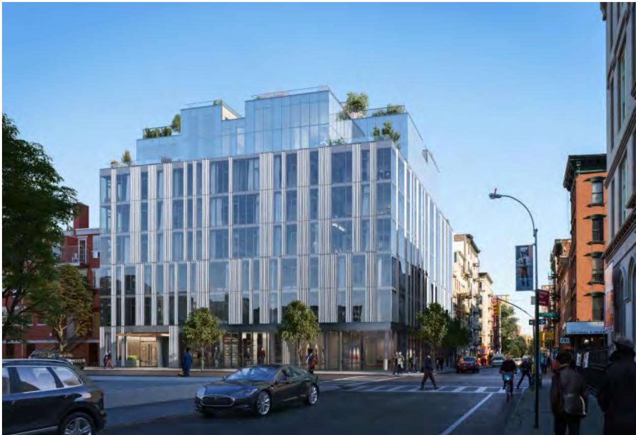
150 Rivington Street. Renderings by GLUCK+. Images via Relevance NY unless noted otherwise.
