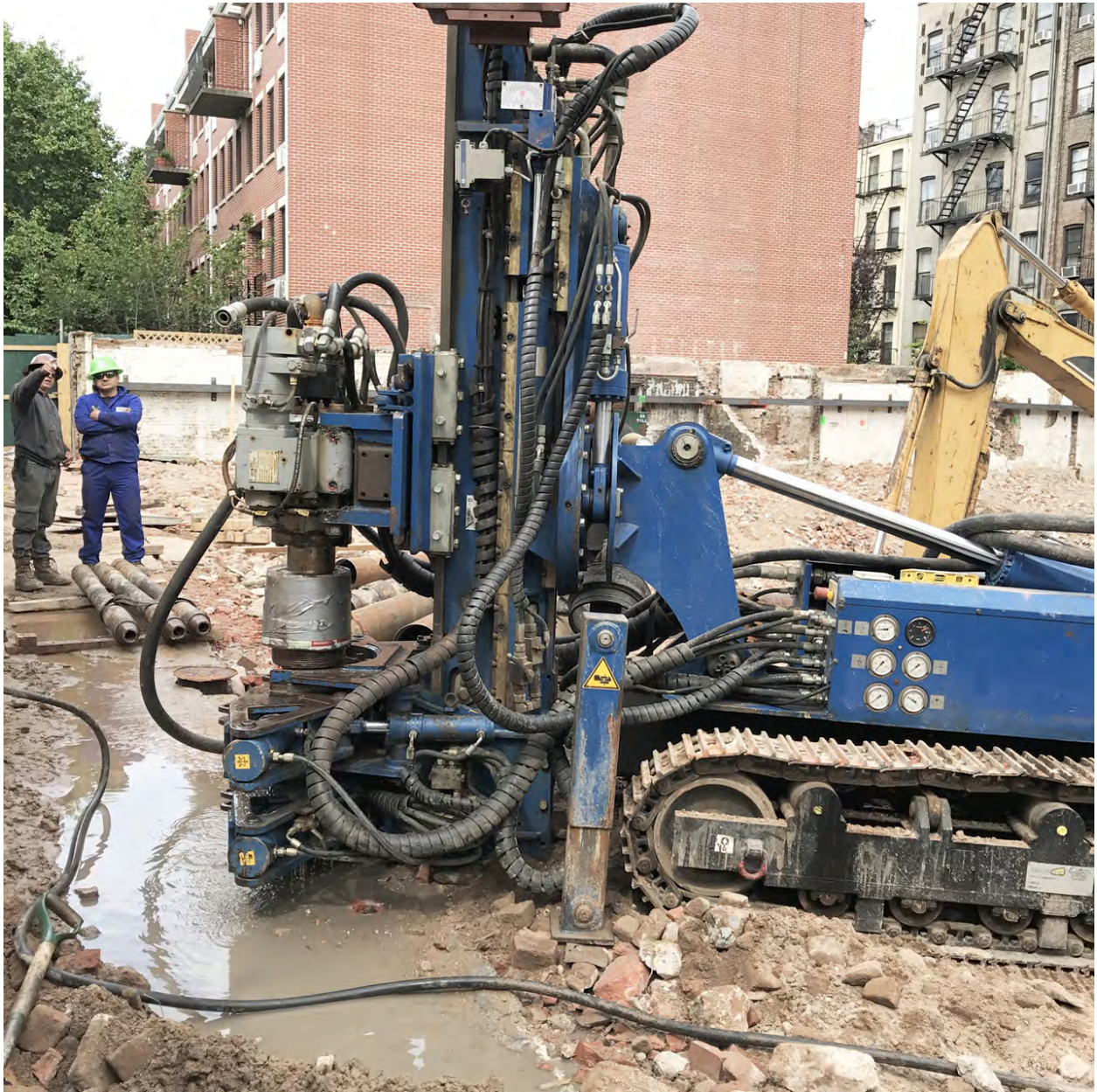
Pile driving at the site.
