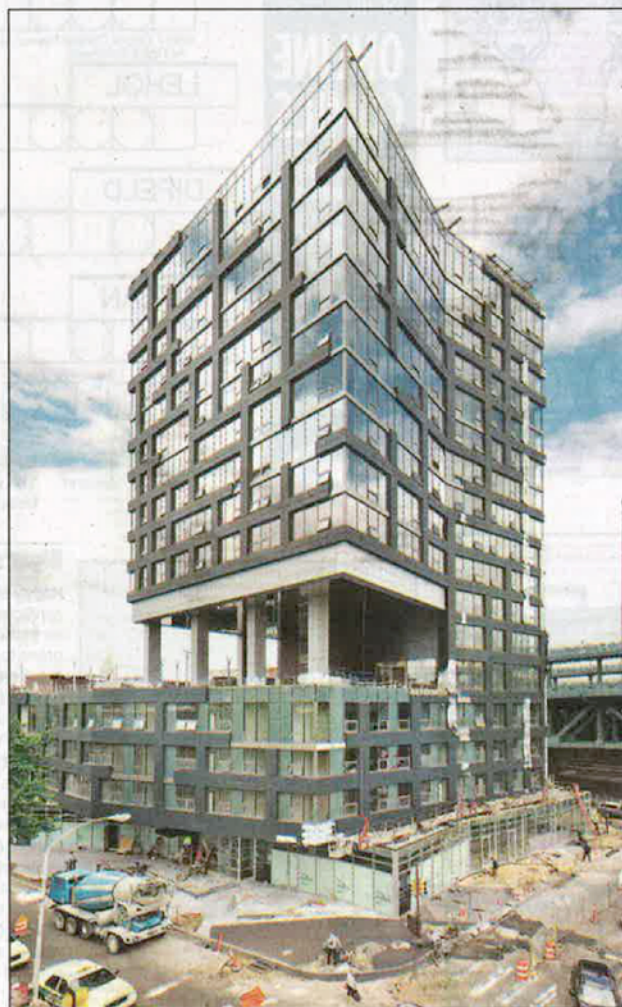
The Bridge under construction at Second and Race Streets. The developers and their architects deserve credit for civilizing this harsh corner and reeling the intersection back into Old City. GLUCK+
