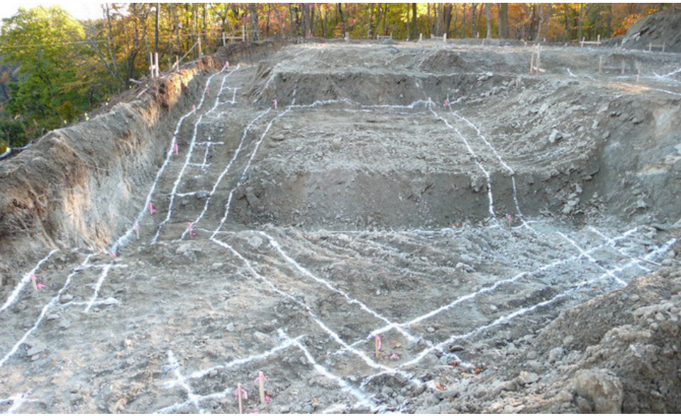
Left: Excavation layout spray painted on site by GLUCK+
