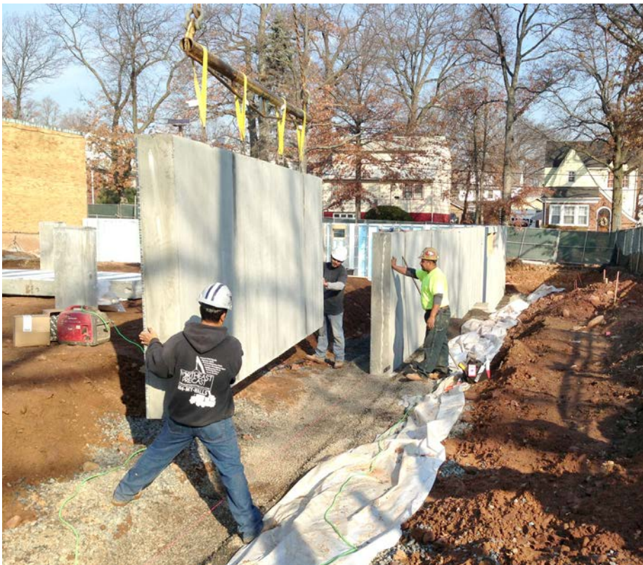
The precast elevator pit and foundation walls—fabricated entirely off-site—were key to meeting the deadline, turning even the foundations into a prefabricated system.
