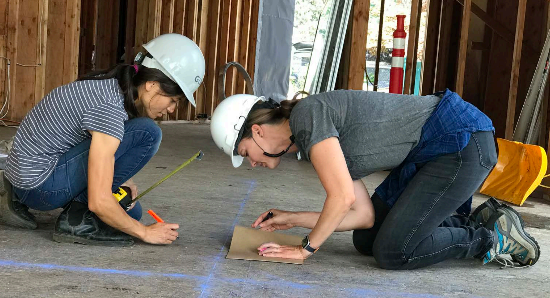
GLUCK+ assists electrical subcontractor with light fixture layout to coordinate with other MEP trades
