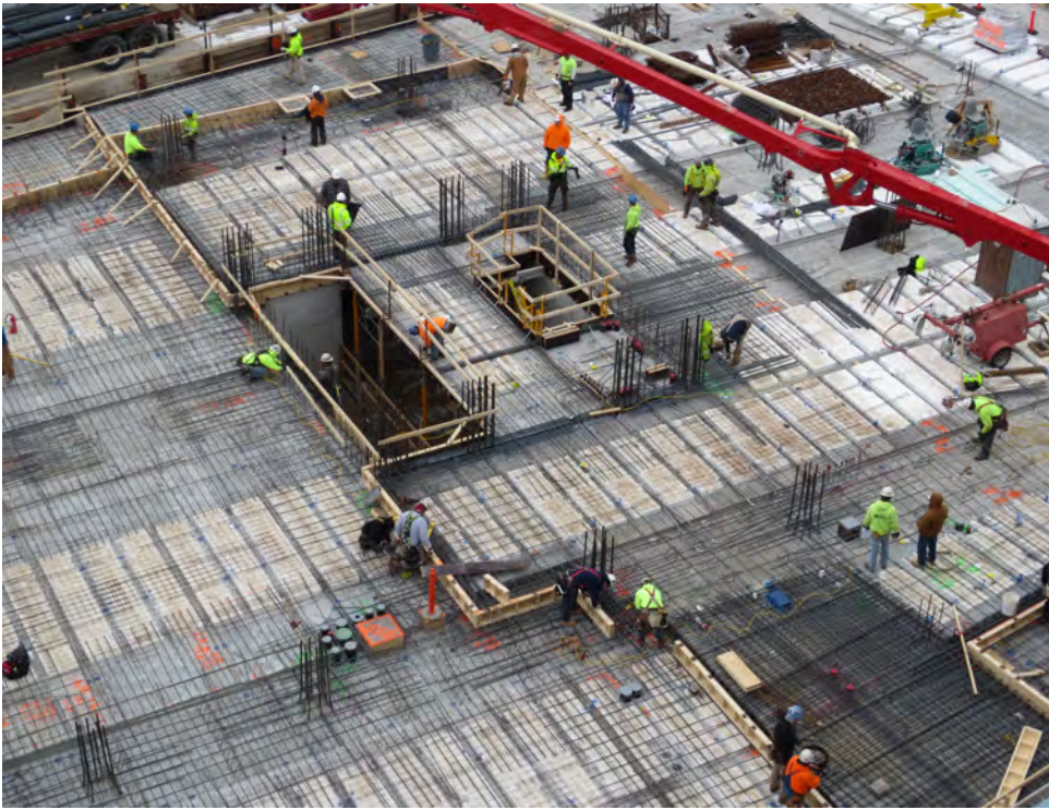
The appropriate system achieves the best building possible, cantilevering the concrete structure and opening the corner views.
