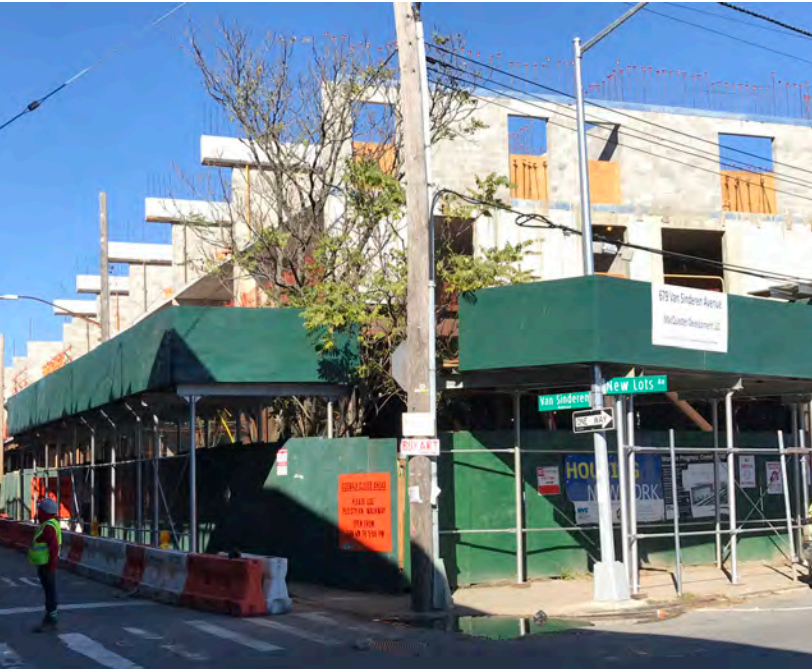
Construction sequence from left to right: 1. CMU bearing walls and concrete beams 2. Cantilevered structure 3. Installation of precast hollow-core planks at the fourth floor
