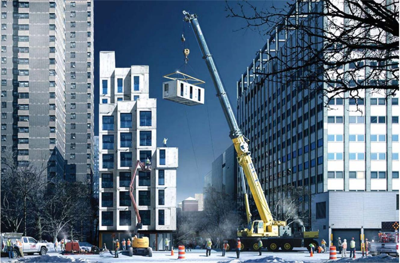
**Figure 1.** Carmel Place is a micro unit apartment building, designed by nArchitects and built in modules, that was commissioned based on winning a competition. (Image courtesy of MIR | nArchitects. Reproduced with permission.)
