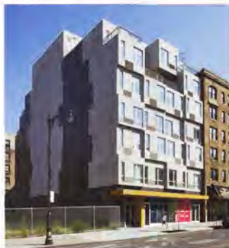
INFILL SITE The seven-story Stack's 56 modules went up in four weeks. The speed could have been increased were it not for transportation restrictions across the George Washington Bridge.
