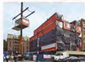
INFILL SITE The seven-story Stack's 56 modules went up in four weeks. The speed could have been increased were it not for transportation restrictions across the George Washington Bridge.
