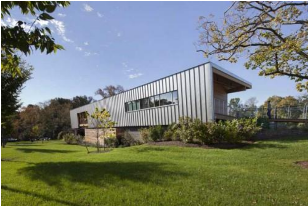
A ZINC ROOF FOLDS DOWN THE BACK OF THE CORDISHI FAMILY PAVILION. (COURTESY VANNI ARCHIVE)
